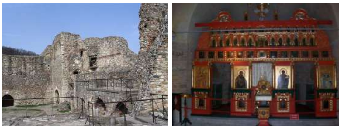
Figure 3: St. Nicholas Chapel (left—before the restoration; right—the altar in the Chapel after restoration)
